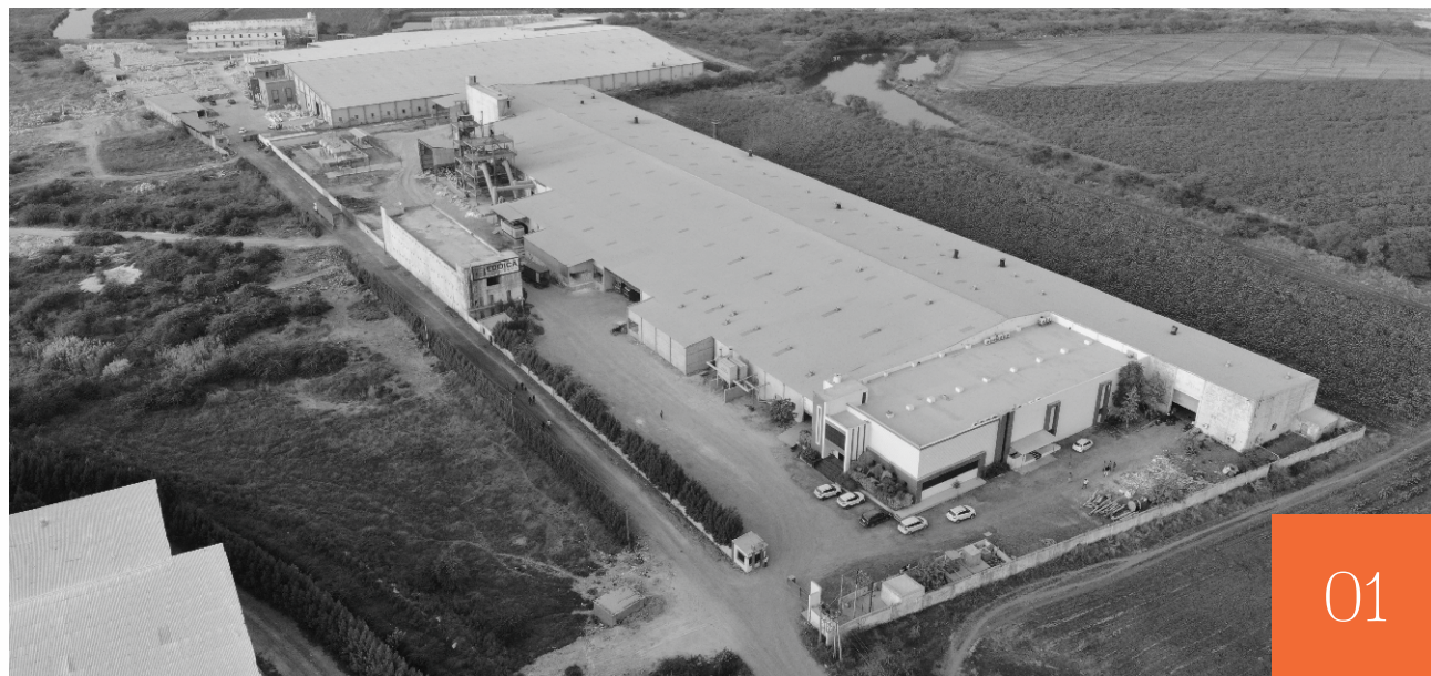
EXCLUSIVE TILES FACTORY
